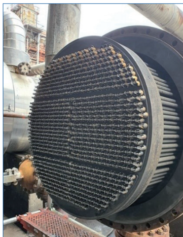
Figure 2 Spirelf on a tube bundle
